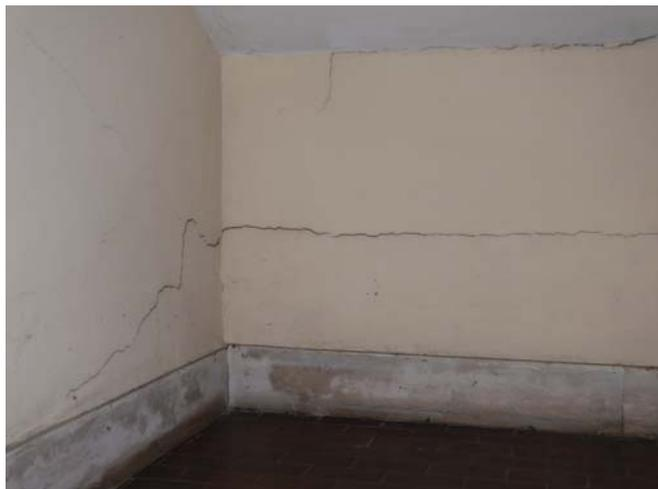
**FIGURA 6** - VIA VOLTERRA 26. APRILE 2010. LESIONI SUI MURI DELLA SCALA A PIANTERRENO. LESIONI NEGLI STESSI SITI ERANO PRESENTI ANCHE NEL 2001, MA SI NOTA NELL'INTERVALLO UN INCREMENTO, SEPPUR LIEVE, DELLE APERTURE
