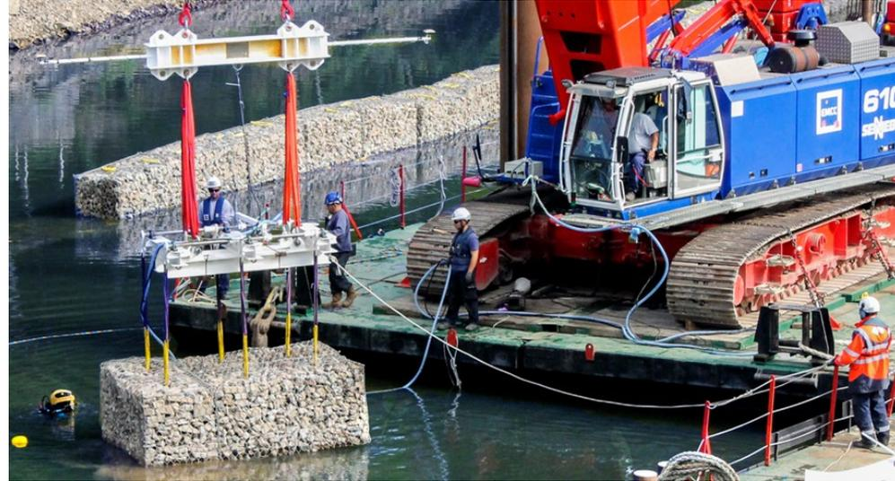
Manufactured with a bigger wire diameter, to provide a higher grade of strength in the hexagonal **double twist wire mesh** ( $\varnothing 3.4 \text{ mm}$ ), due to the high stresses during handling operations (lifting & launching)
